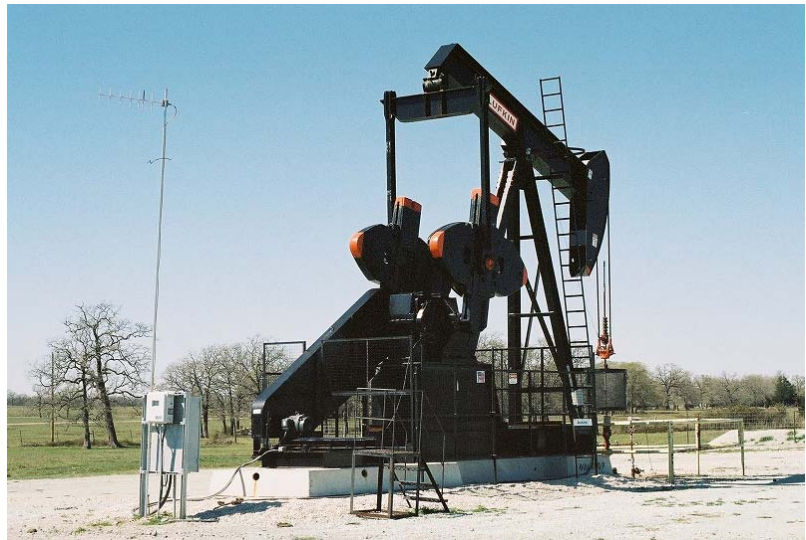
A pump jack near Houston.
