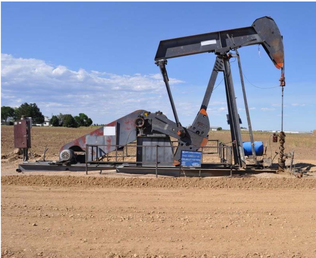
Pumping station outside Denver, Colorado Photo by Flow Research
